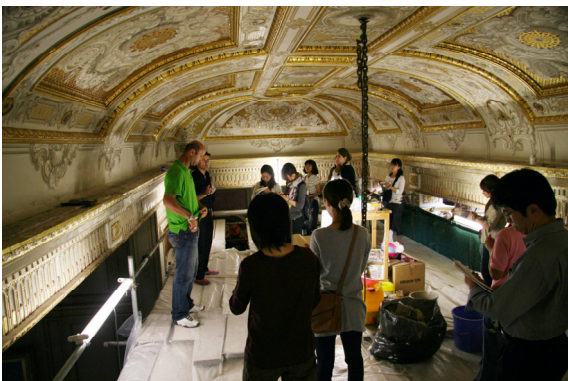
Site visit to an ongoing restoration in the Dolmabahçe palace
